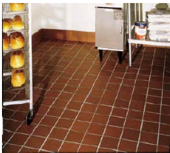
After 14 days, a significant improvement in the grout's colour.
